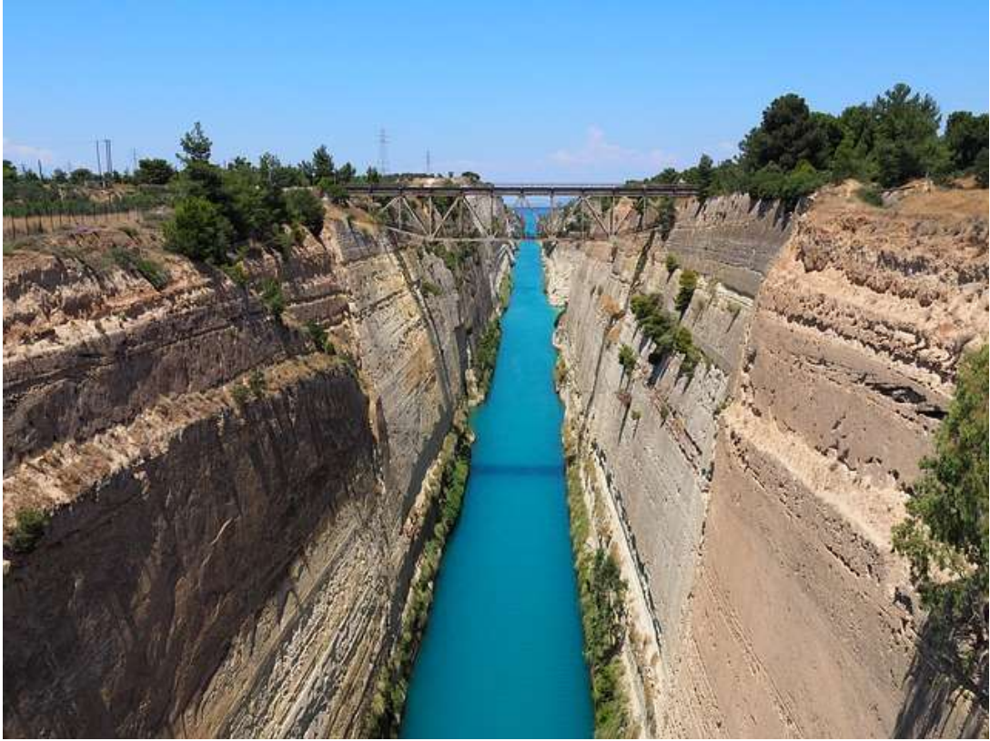
Figure B4 Present-Day View of the Corinth Canal
